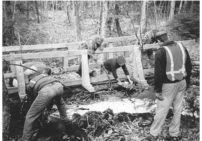
Working to Reset One of the Kilburn Brook Bridges
